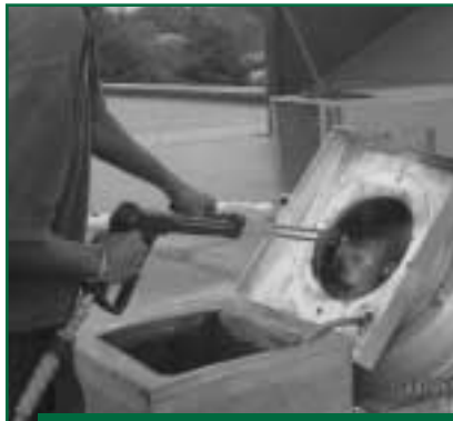
Technician pressure-washing a rooftop fan
